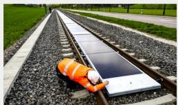
Swiss start-up Sun-Ways installed 48 test solar panels between train rails, producing 16 MWh/year (4-6 homes). More panels can be placed or removed in a few hours for easy maintenance and cleaned by passing trains to generate 2% of grid power from 5,320 km of Swiss rail (1 billion MWh/year, 300,000 homes). Stations and platform roofs can also be used.
