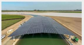
A \$20 million, 1.6 MW solar array now covers part of the Turlock Irrigation District canal system in California's Central Valley, providing power to farmers, keeping panels cool, and limiting evaporation in drought-prone areas. 8,000 miles of federally owned canals and aqueducts coul
