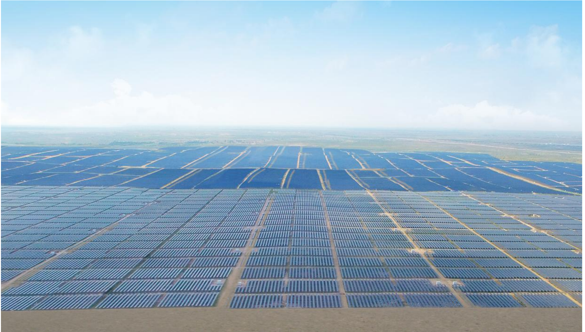
1-GW Yanchi PV solar plant in Qinghai, China
