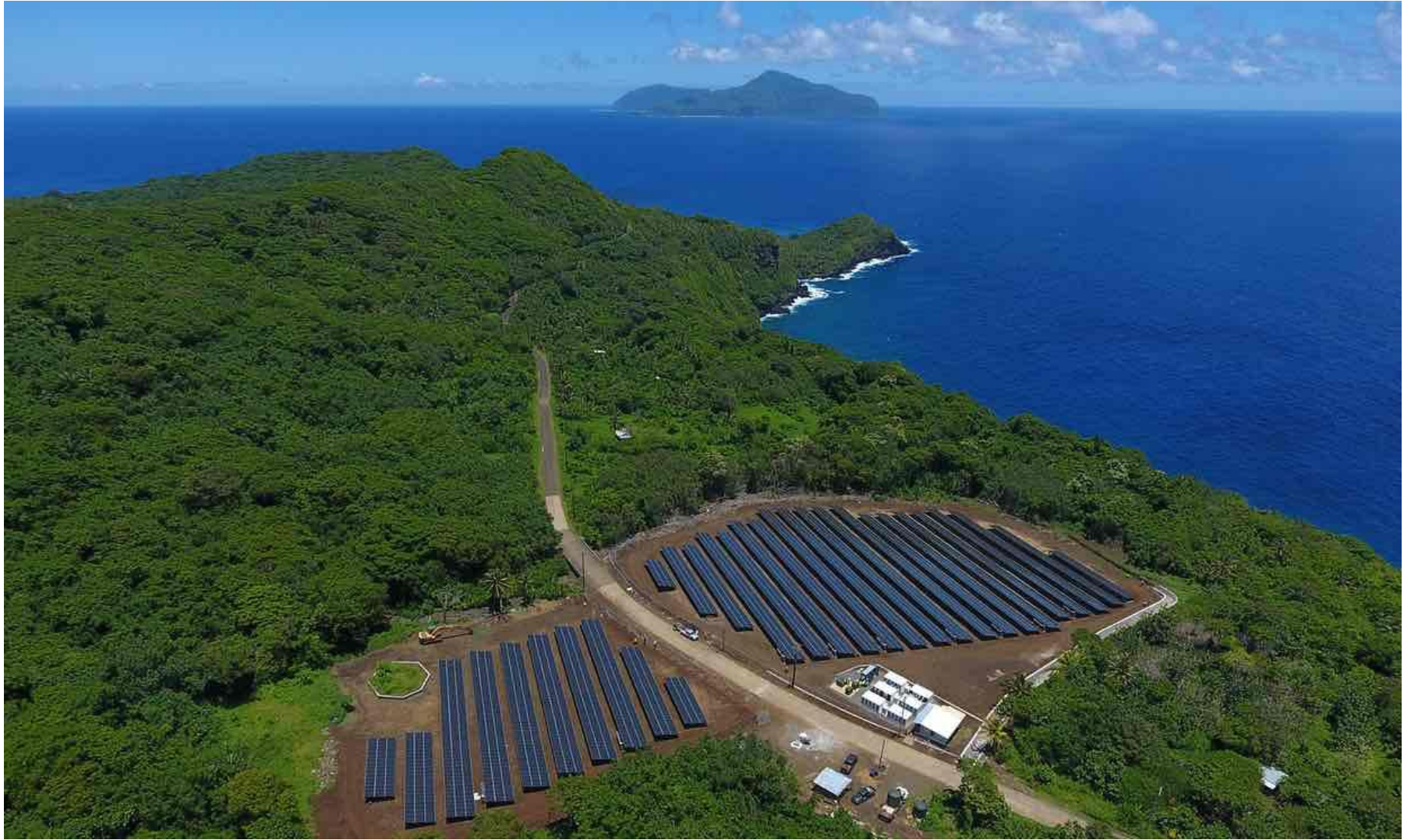
American Samoa: Photovoltaic
