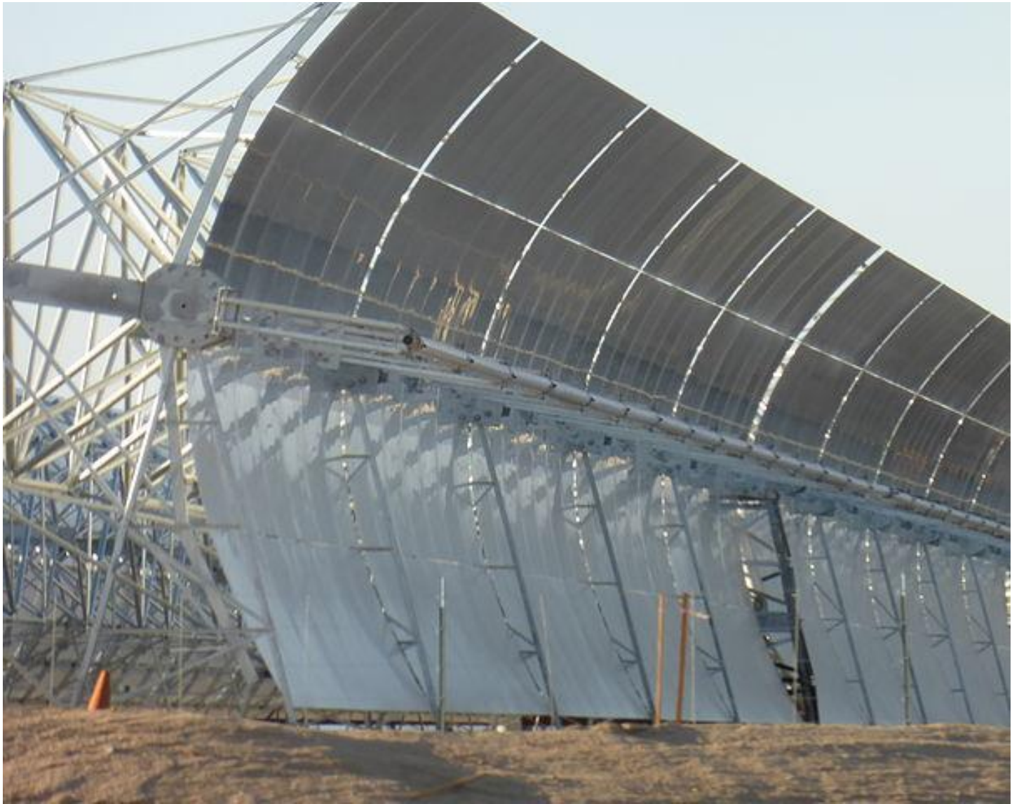
Noor1 Morocco – parabolic trough
